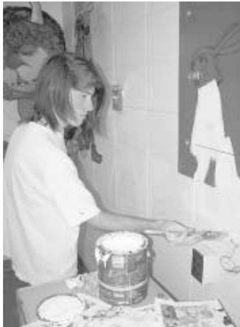
Kenneth Shearer works on the entryway to the school's library.
